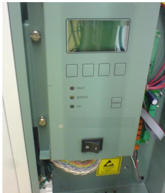
Figure 2: Humidifier Keypad / Front of PCB
