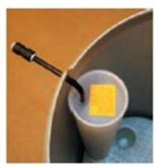
10. The system is now ready for start-up NB! There must always be a floor drain to avoid damage caused by leakage.
