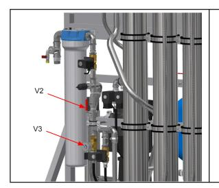
Open both the recirculation valve (V2) and the outlet valve (V3)\*
