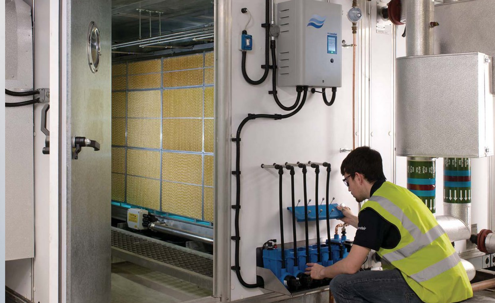
Nortec ME with externally mounted hydraulic unit
