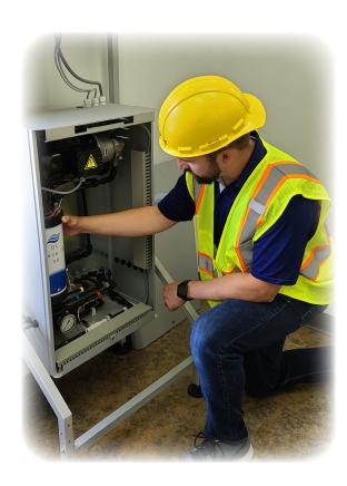
Wear and tear can affect the performance of any humidification system. Preventive maintenance can go a long way to optimize production time by addressing potential problems before they become costly emergency repairs.
