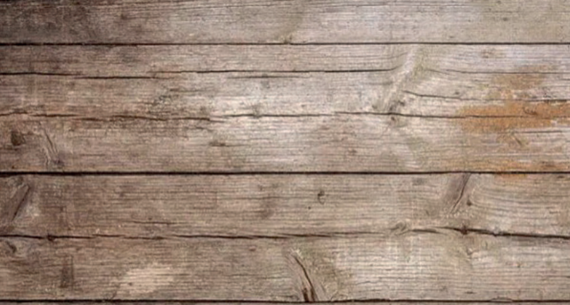
Hardwood floor cracking due to low air humidity levels.
