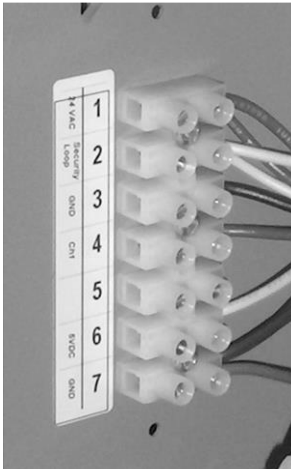
Figure 13: Low voltage terminal strip on NHRS Humidifier
