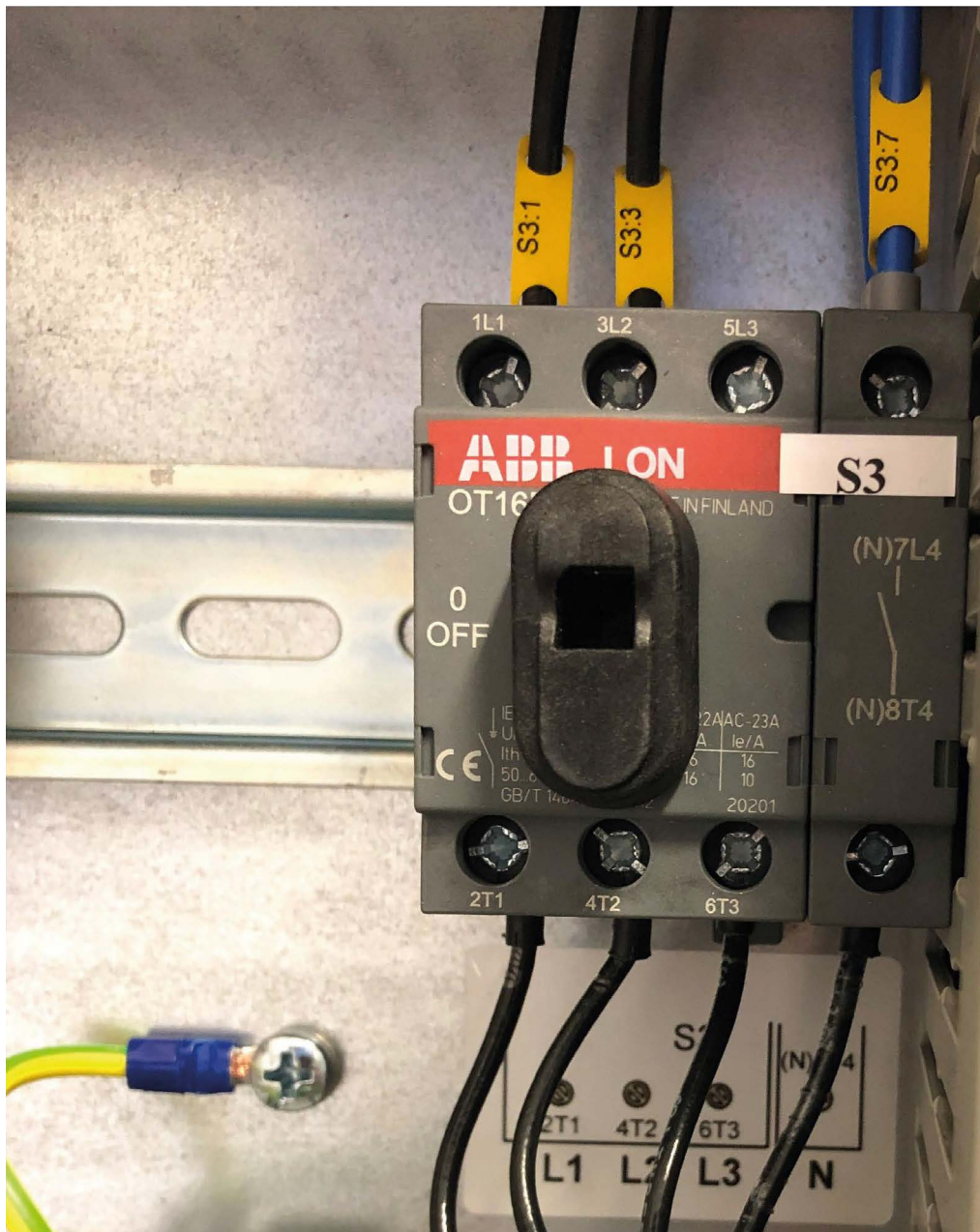
Fig. 52: Connecting the power supply
