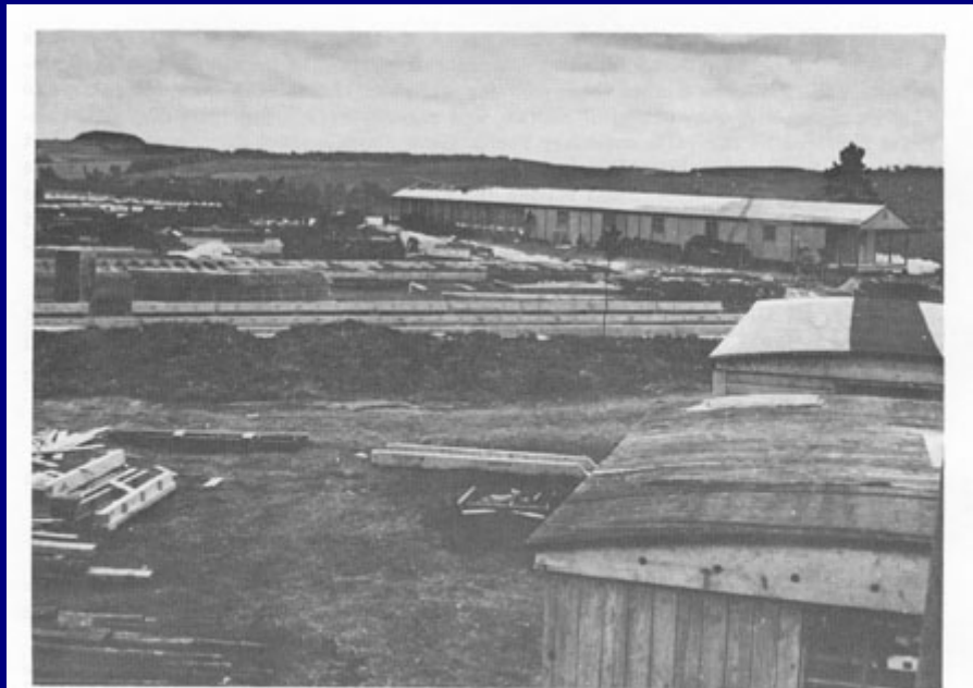
FIGURE 45.—The American Red Cross-Harvard Field Hospital Unit, assembled in Salisbury, England, from 66,000 pieces of prefabricated building material shipped from the United States. The hospital was used to study wartime epidemics. (Photograph, courtesy American Red Cross.)
