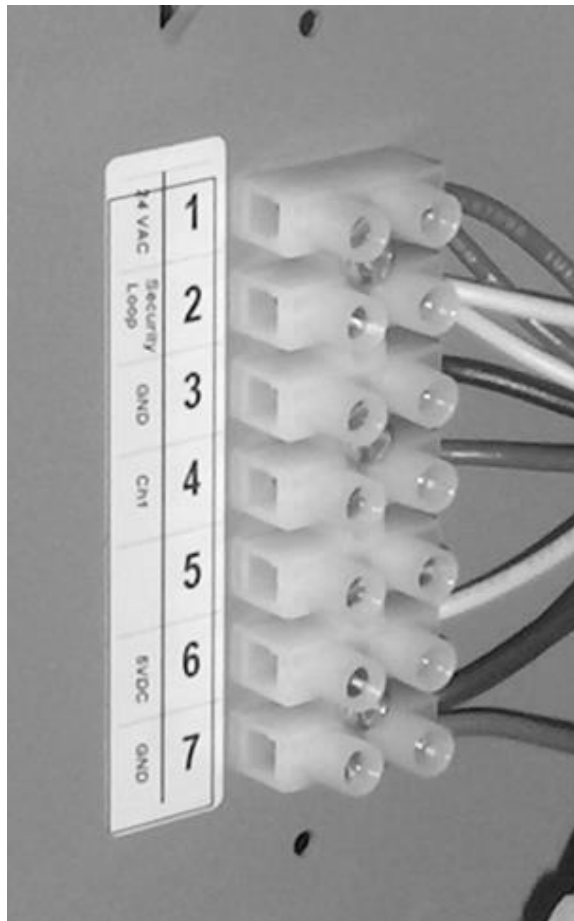
Figure 13: Low voltage terminal strip on Nortec NHRS Humidifier
