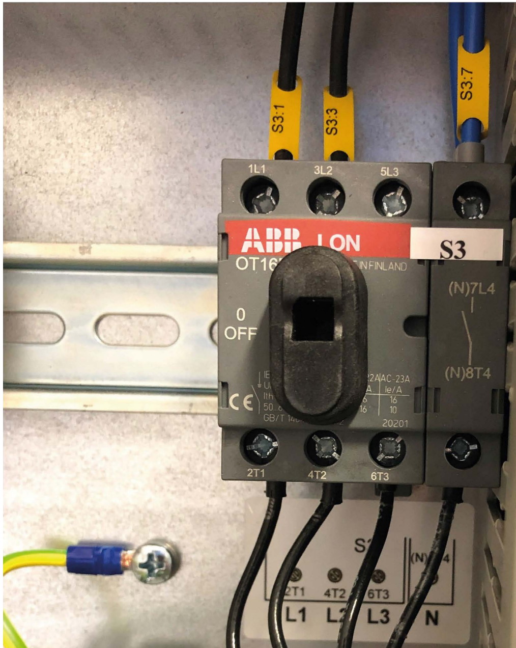
Fig. 52: Connecting the power supply
