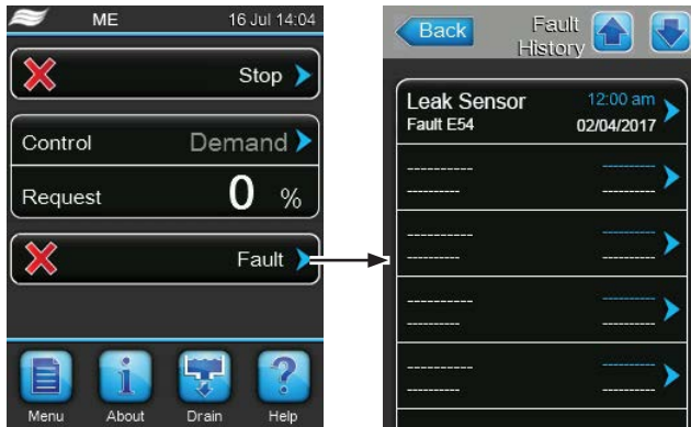
Fig. 3: Fault indication on display
