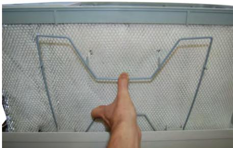
Fig. 28: Remove filter bracket
